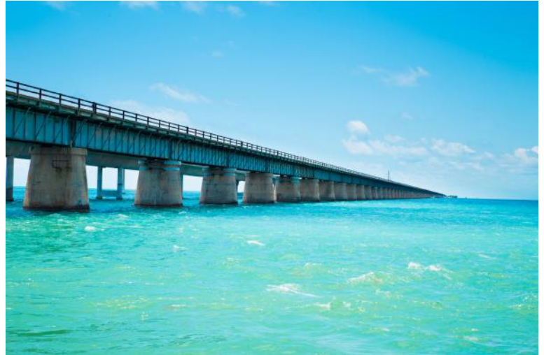
The 7 Mile Bridge in the Florida Keys is an example of a beam bridge.
