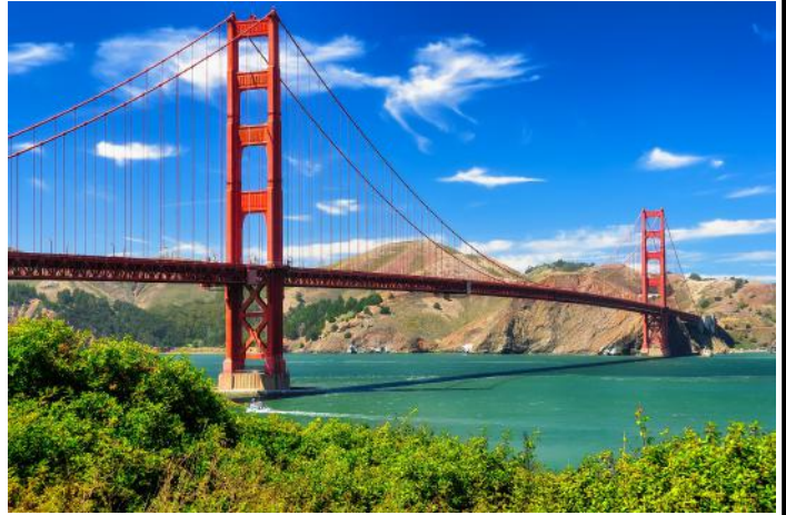
The Golden Gate Bridge in San Francisco is an example of a suspension bridge.
